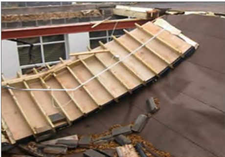
What can happen when a roof is subjected to excessive loads from ponding of rainwater
