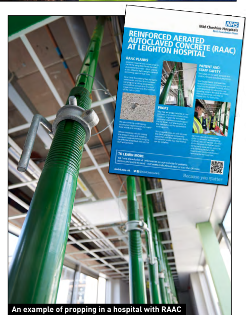
An example of propping in a hospital with RAAC
